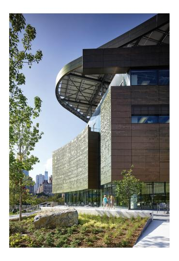
The digital patterning of the perforations was created by running the rainscreen panels through a repurposed welding robot. Students from Cornell Tech and the Massachusetts Institute of Technology (MIT) collaborated with Zahner to develop the algorithm that controlled the device, which made them major contributors to the façade design.
