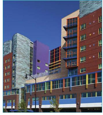
**Coraflon** and **Duranar** fluoropolymer coatings were specified for their low maintenance requirements, increased durability and color retention. The **Coraflon** coating colors shown here provide bright and vivid colors on the exterior of Children's Hospital.
