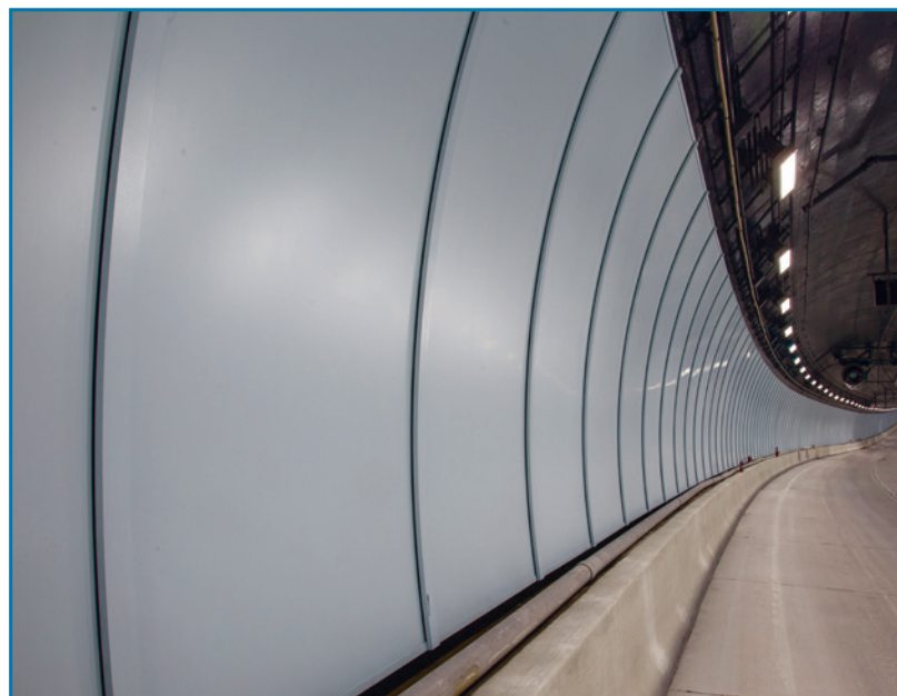
The 4,000 solid aluminum plate panels lining the tunnel were painted with Duranar XL Crystal Blue coatings, while the lattice work was coated with durable Duracron coatings.
