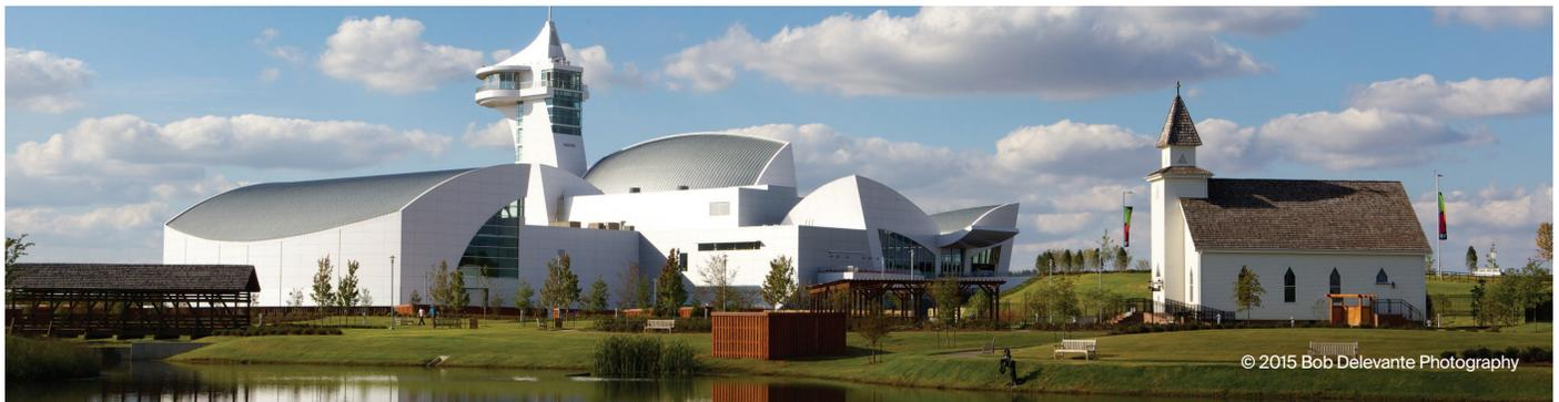
The Discovery Center is the cornerstone of Discovery Park of America, which was built on a former 50-acre cornfield. The structure’s futuristic-looking exterior is finished with Pure White *Duranar* coatings and Bright Silver Metallic *Duranar* XL coatings by PPG.
