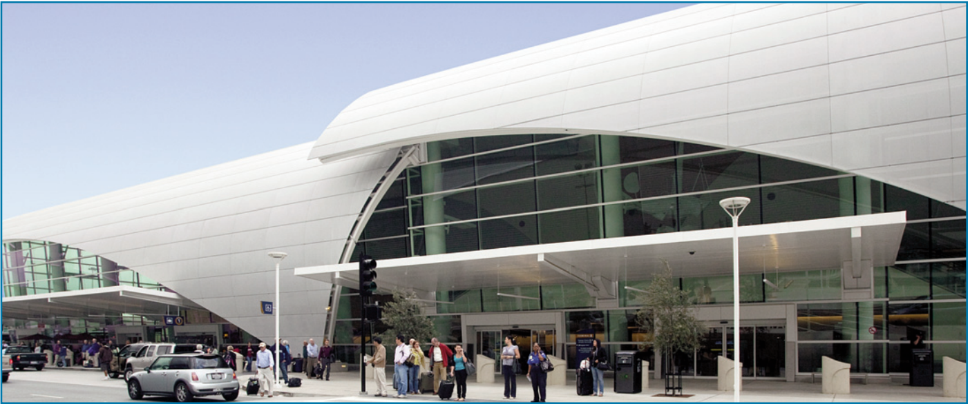
Duranar powder coatings in Regal White coat the perforated panels that envelop San Jose International Airport's Terminal B.
