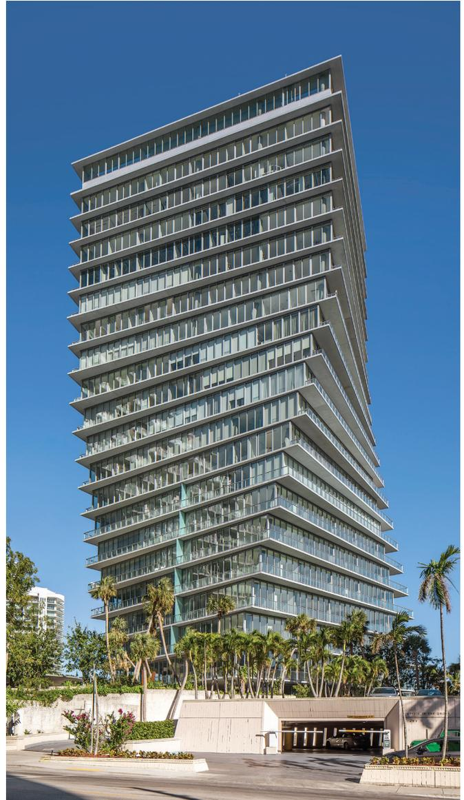
Tecnoglass selected *Duramar* coatings for the Grove at Grand Bay because they offer the proven seacoast corrosion performance required for projects in humid, salt-air environments.
