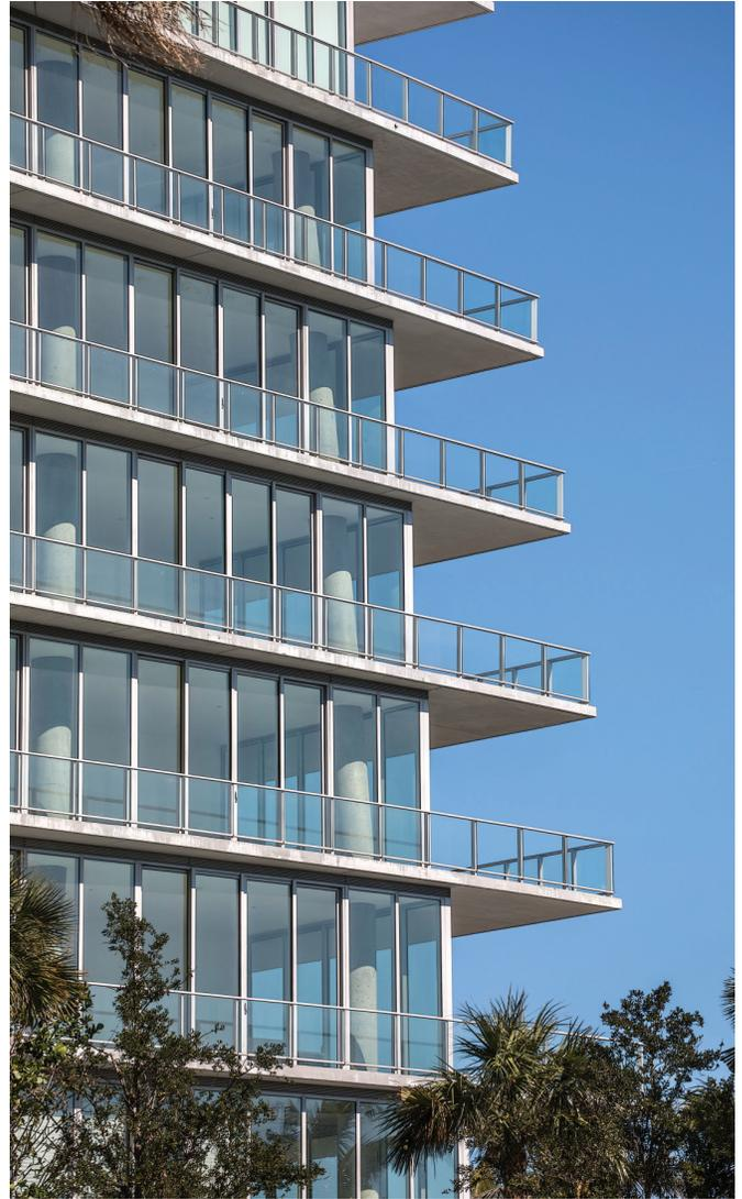
Tecnoglass, a PPG Certified Applicator Program member, engineered hurricane-resistant window walls, glass doors and metal framing systems finished with *Duranar* fluoropolymer coatings by PPG.
