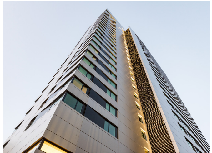
The House at Cornell Tech features two custom-formulated PPG Duranar MXL coatings, including one called Zenon Atoms, for the building skin. The coating color-shifts from a silver to champagne color in response to changing light conditions.
