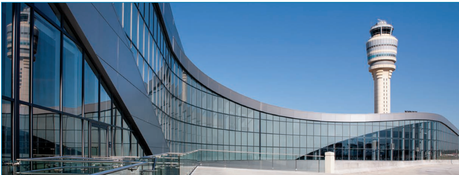
Duranar ® XL 70-percent fluoropolymer coatings cover nearly three-quarters of the exterior curtain wall. The coatings are exceptionally flexible and highly resistant to abrasion and chipping, helping the panels to maintain their original appearance over the years.
