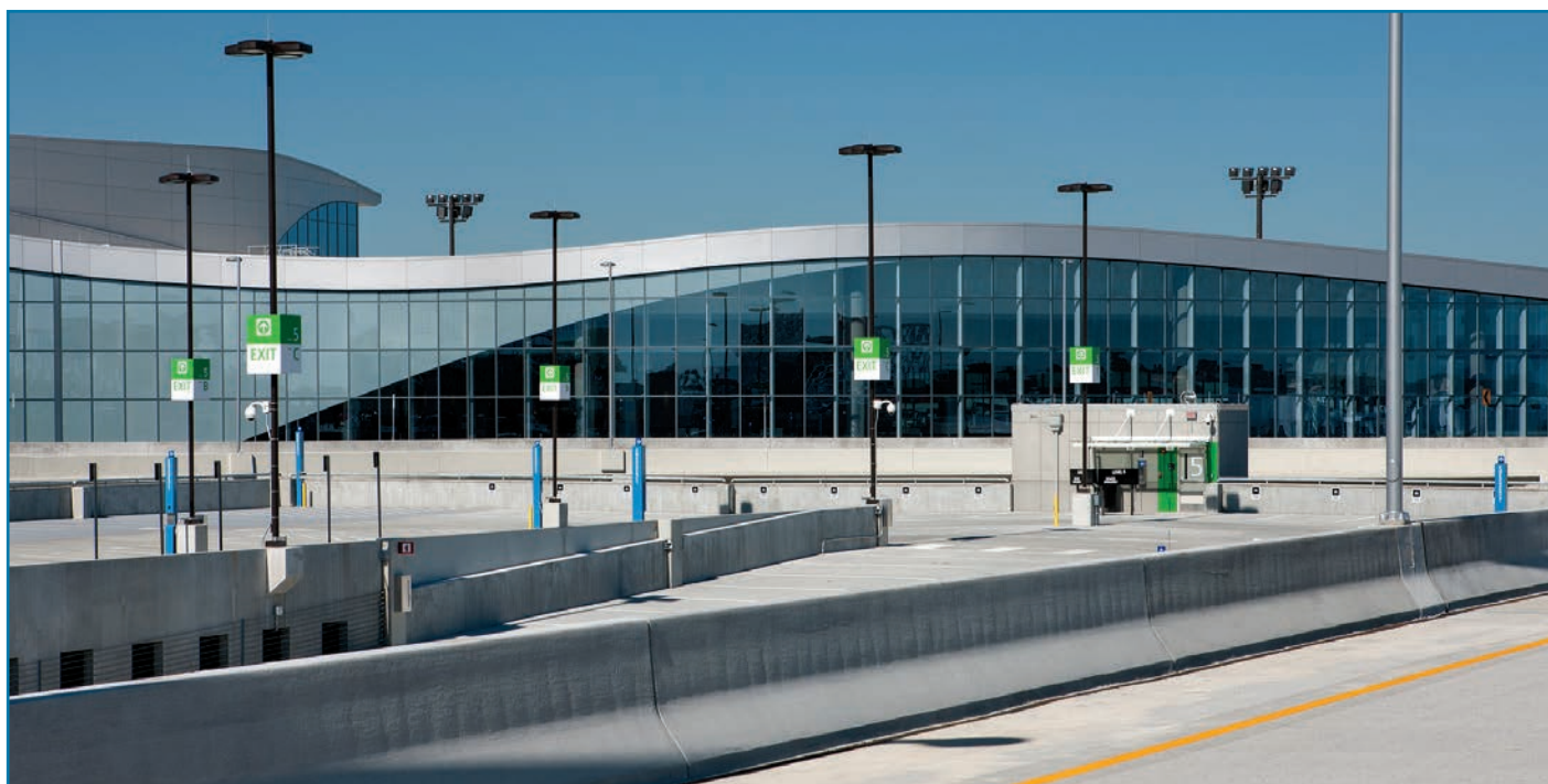
The exterior curtain wall of the Maynard H. Jackson Jr. International Terminal features 264,000 pounds of aluminum extrusions painted with Duranar XL coatings by PPG.
